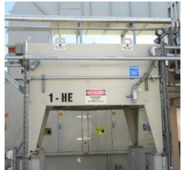
Air exchange (fin/fan) oil cooler
