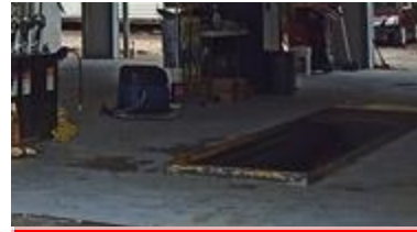
Non-Compliant Service Bay
